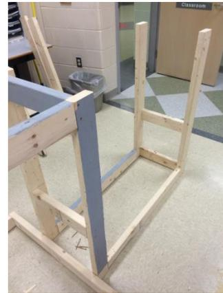
9. Cut two horizontal supports of 42" each (out of 2x4)
